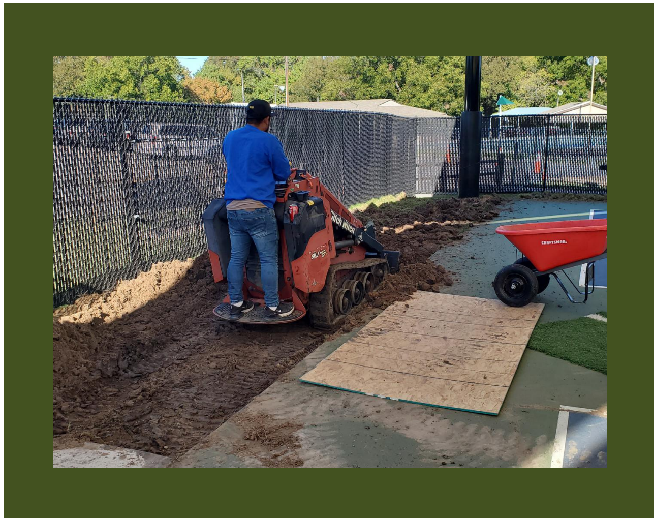
HARRY MYERS PICKLEBALL COURT ARTIFICIAL TURF INSTALLATION
